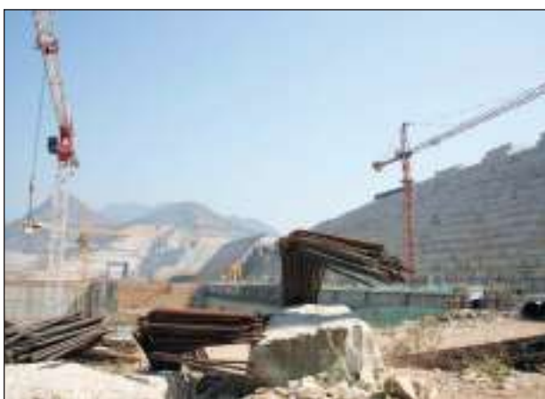
The construction site of the dam
