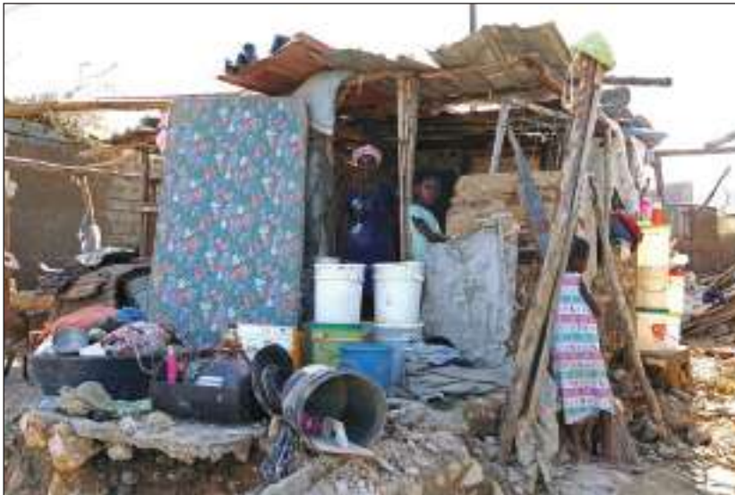
Photo 5.5 – Damage to housing
